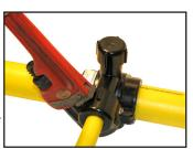
**5** Screw punch down until stop on drive key contacts the top of the saddle tee. The tap is now complete.
