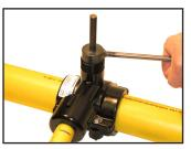
outlet. Do not overtighten. **CAUTION:** To prevent inadvertent pull-out of the P.E. tubing during the assembly process, complete step 11 immediately after step 10, without delay and ensure work is not being performed on the free end of the P.E. tubing.
